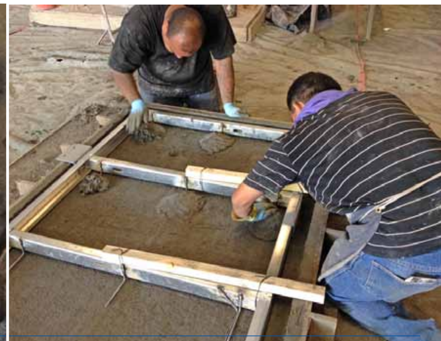
Pre-engineered panels with anchors embedded in the cast simplifies installation.
