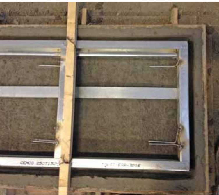
Pre-engineered panels with anchors embedded in the cast simplifies installation.
