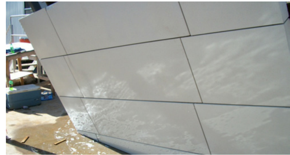
Fabrication – Finish Mock Up
